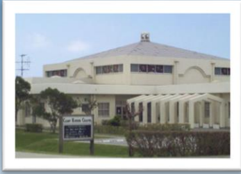
CAMP KINSER CHAPEL BLDG. 1092 Phone: 637-1148
